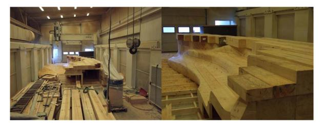
The whole structure was transported by semi-truck from the factory to site in 3 large pieces and placed into the steel and glass frame. The wood is assembled in a traditional way using only wood pegs as fasteners. Finally, the surface is polished by hand machines, and all edges are processed with traditional hand tools. The south facing exterior wall is treated with pine tar while the interior wood has been oiled.
